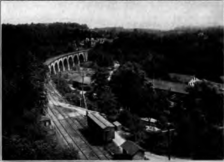
THE FAMOUS THOMAS VIADUCT, ON THE BALTIMORE & OHIO AT RELAY, MD., BUILT BY B. H. LATROBE IN 1835, AND STILL IN USE
